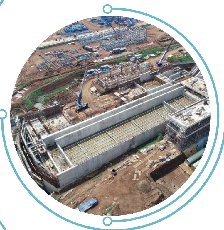
Aeration Basin Reinforcing bar, Formwork, Concrete pouring, Piping Work
