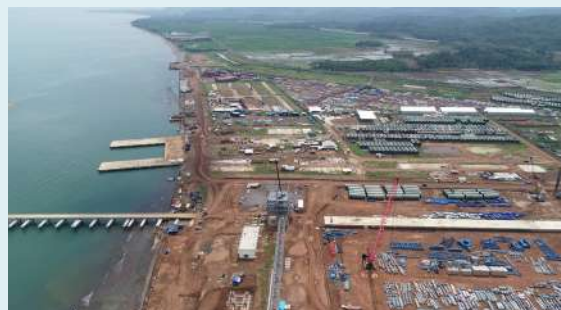
Pemasangan Pengaman Pantai Sementara The Installation of Temporary Shoreline Protection
