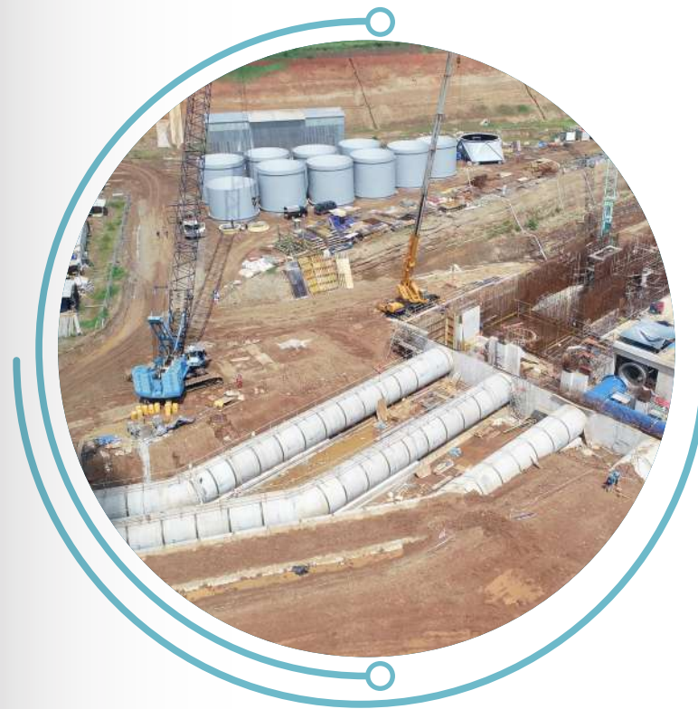
Intake Pond Reinforcing bar, Formwork, Concrete pouring, Piping Work
