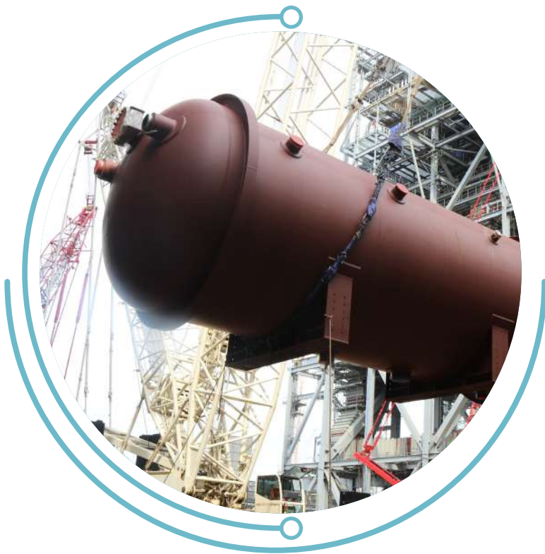
Deaerator Unit # 1 Lifting and Setting Deaerator
