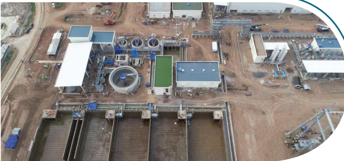
○ Waste Water Treatment Plant Mechanical and Electrical Equipment Installation
