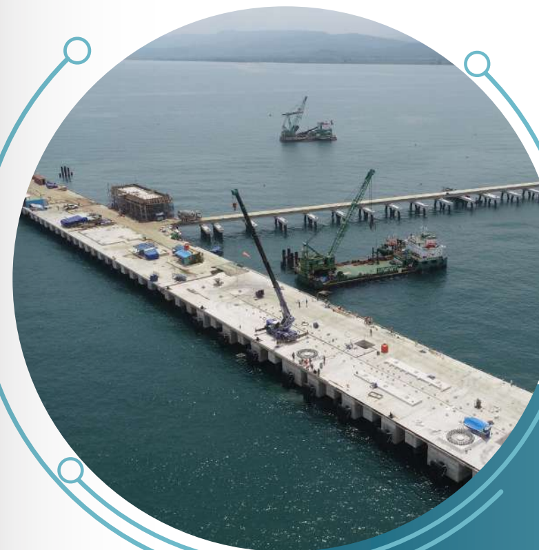
Coal Unloading Jetty Civil/Architectural: Install Fender, Bollard, Handrail, and Electrical Room Mechanical : Install Ship un-loader crane, Conveyor Frame Support
