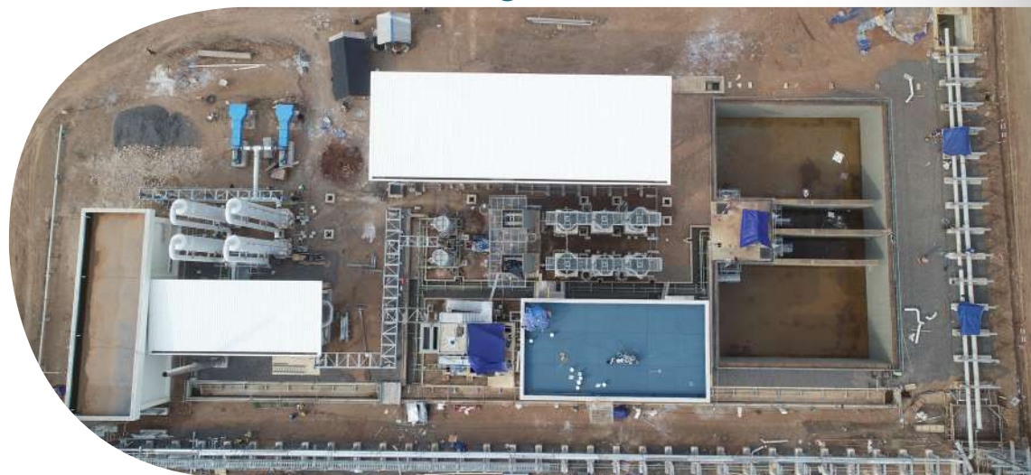
Ammonia Removal Plant ○ Mechanical and Electrical Equipment Installation
