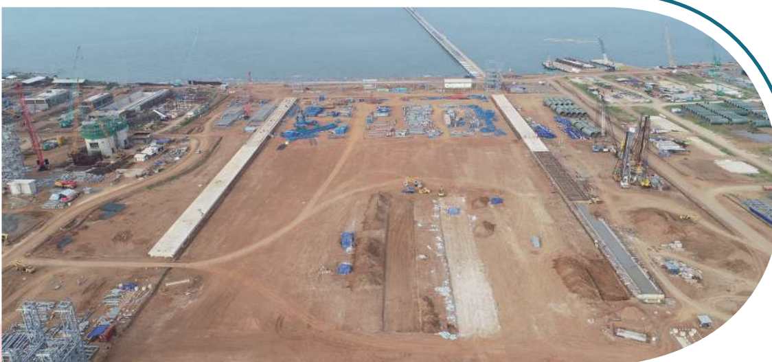
○ Coal yard Cement Shallow Mixing, Concrete Foundation for Stacker Reclaimer and Equipment assembly
